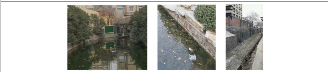
Fig. 4-13 Currently water problems, Photos taken by author.
