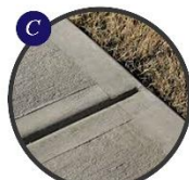
Concrete Expansion Joint
