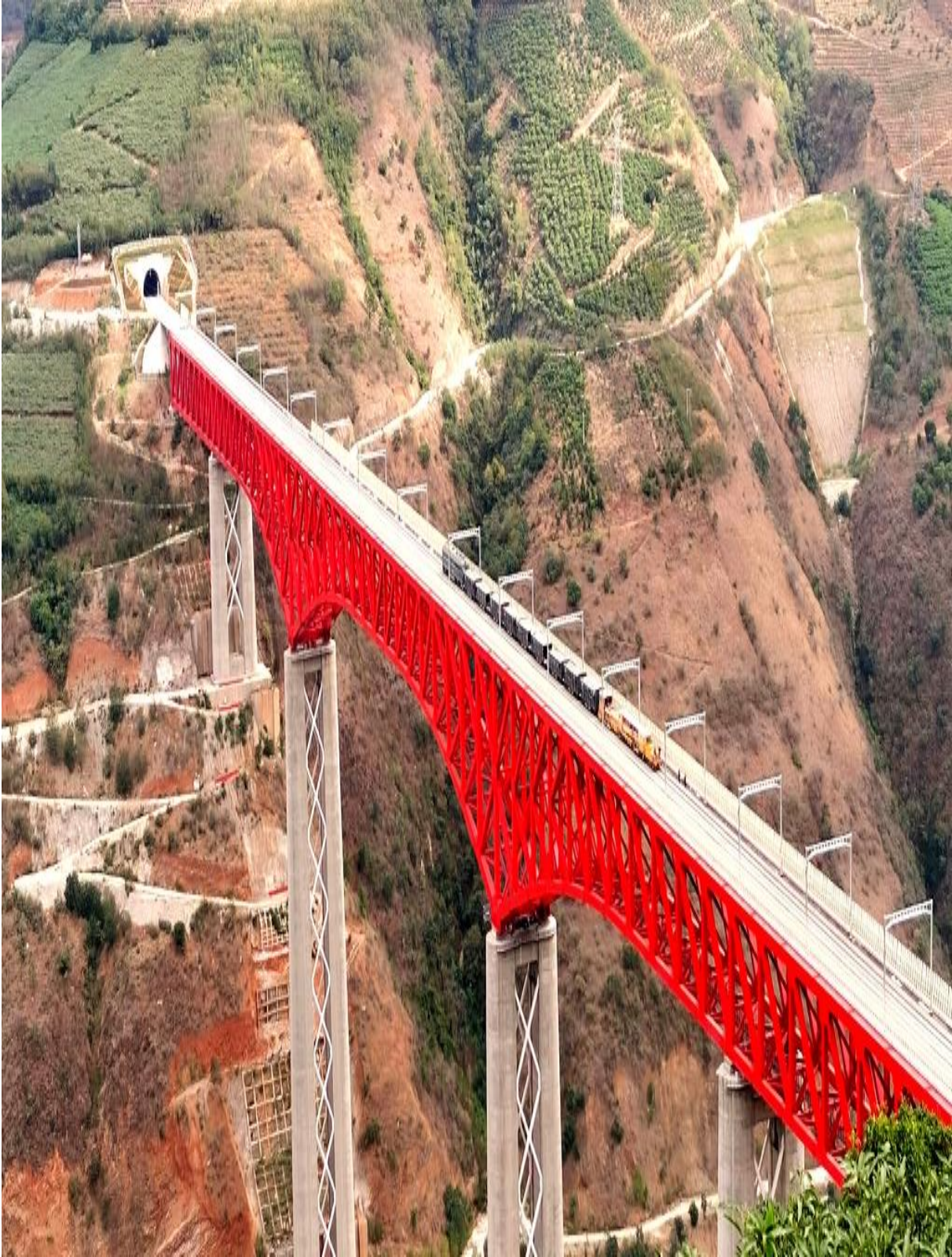
Figure 9: Tunnels and Bridges of Lao-China railway
