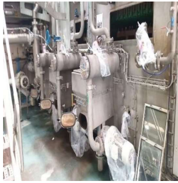
Figure 67 - Filter of the first, second and third bath of the washer.
