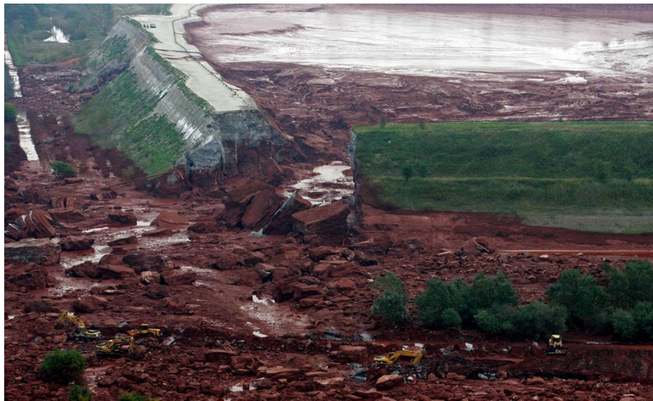
Figure 5: The ruptured wall of a red sludge reservoir 2010, Kolontar Hungary
