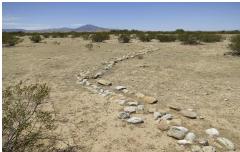
Figure 3. Single rock contour berm, Arizona, USA. (Stavi et al. 2020).
