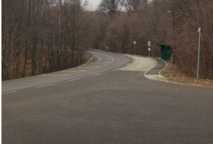
Figure 16. Road infrastructure in Mátra
