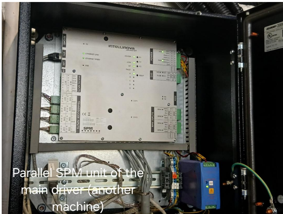
18. Figure: Parallel SPM unit of Main driver (Source: Own photo, Arconic Székesfehérvár plant (2025))
