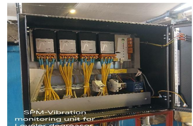
13. Figure: SPM-Vibration monitoring unit for the stretch leveler degreaser (Source: Own photo, Arconic Székesfehérvár plant (2025))
