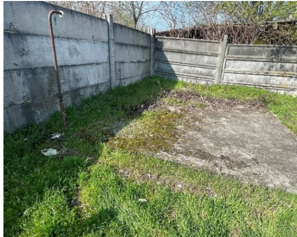
18. ábra – beton platform
