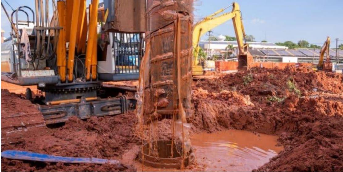
Figure 3: Large diameter second-class well under construction in Morocco (Source: http5 )
