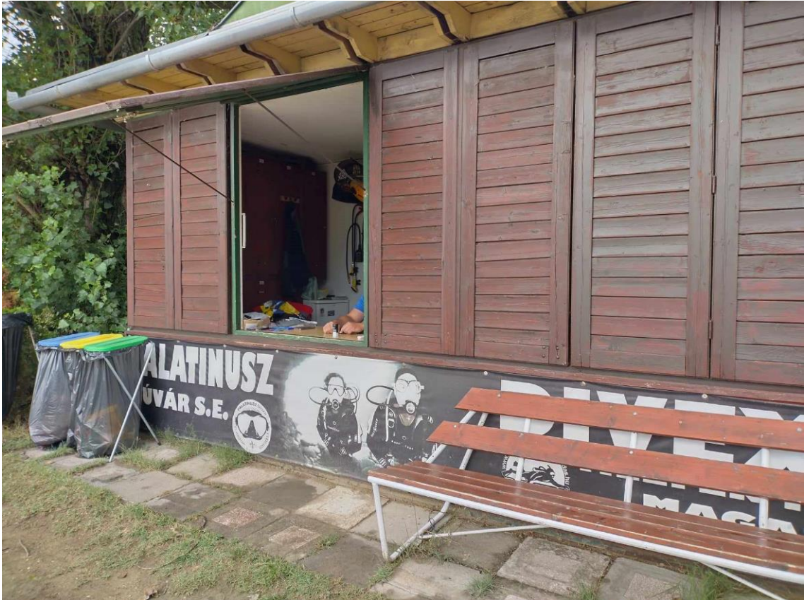
Fig 20: The current state of the base is a mixture of unorganised, differently designed elements
