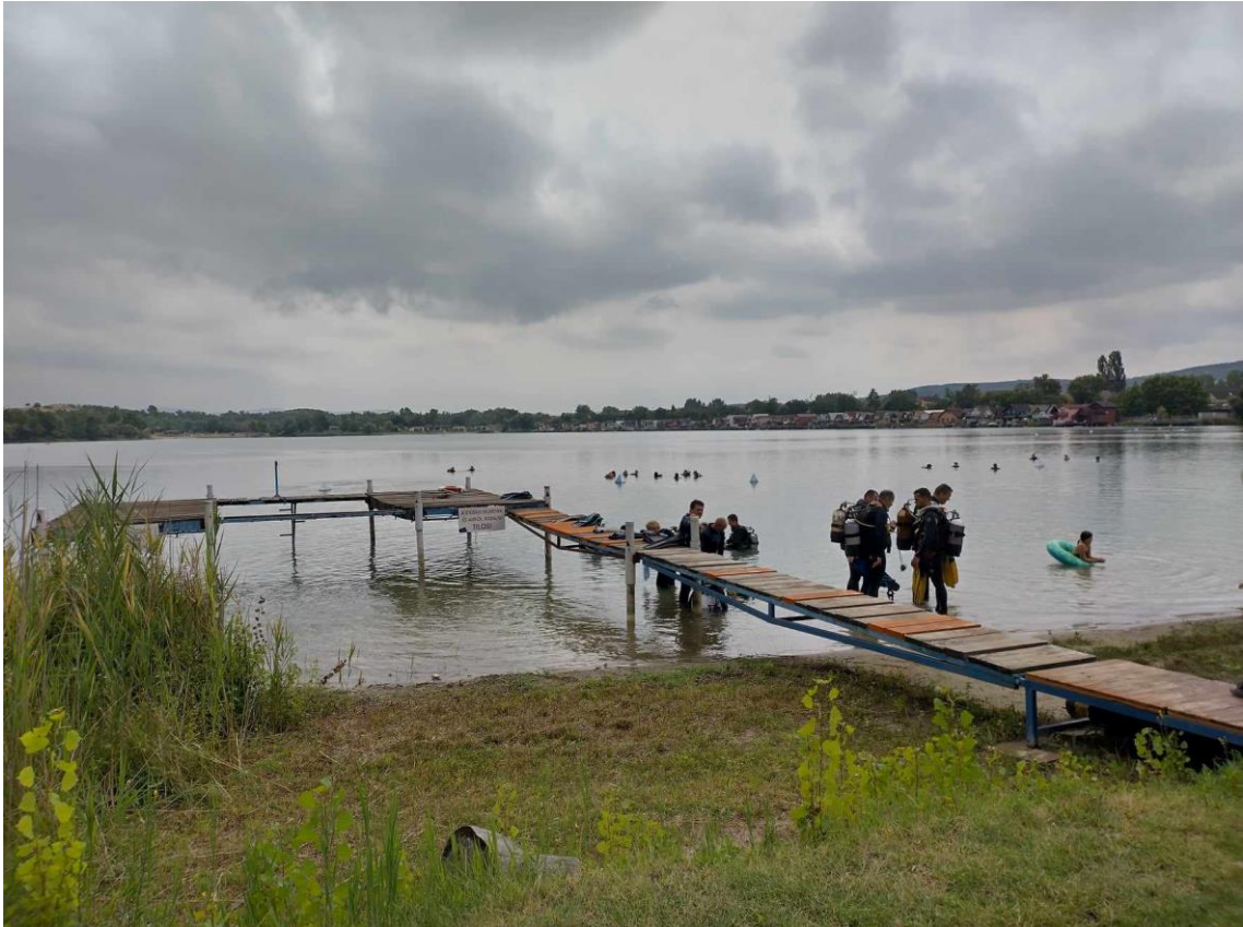
Fig 19: The current state of the wooden deck on location
