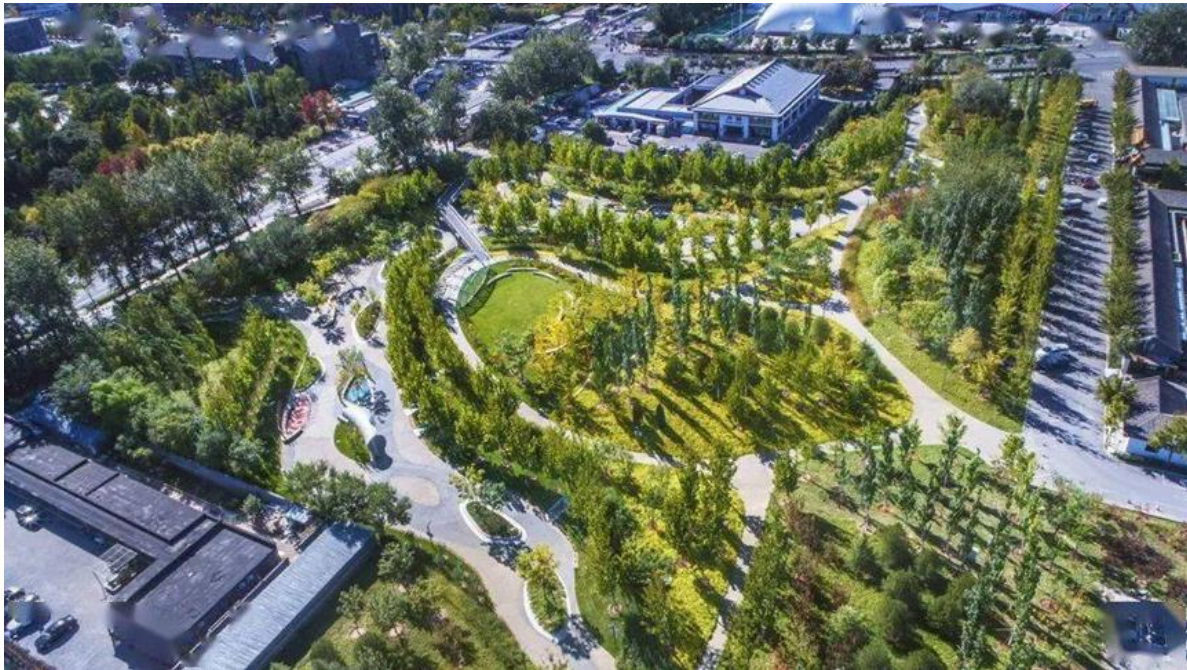
Figure. 5 Aerial view of West Chang'an Street Culture and Art Park /(INT-12)
