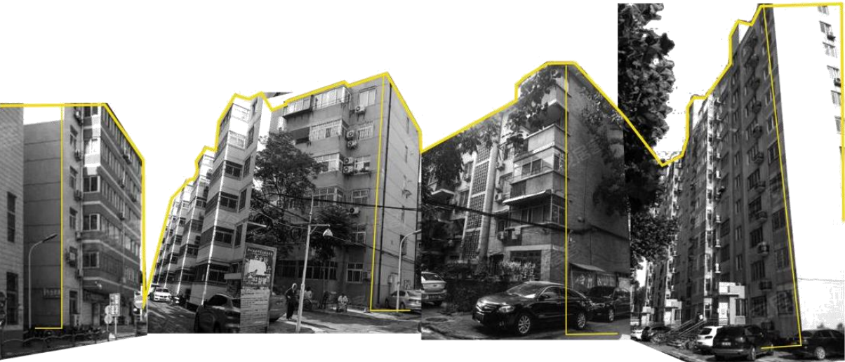
Fig. 2-5 Building photo of the community. Source: by author
