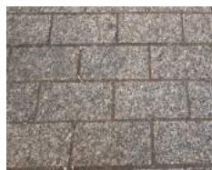
The pavement in the central area
